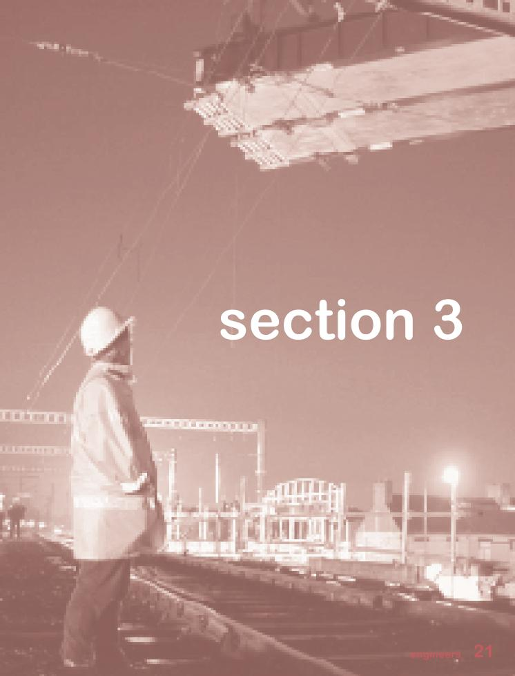
Pic. on previous page: The Big Lift by Paul Wilcock Aug 2002 – Prefabricated East Wall Road Rail Bridge deck being lifted over the Dart line at East Wall into its final position by Demag PC9600 crane.
